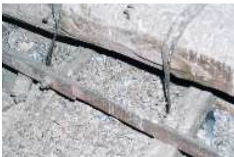
DETAIL OF VAULT REINFORCING
