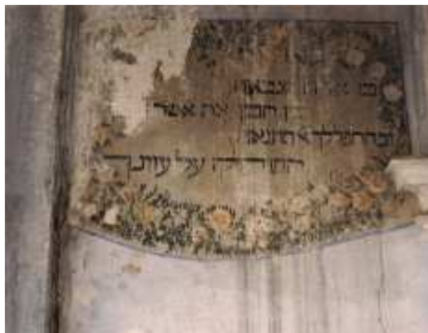
SIGNS OF MOISTURE INFILTRATION
