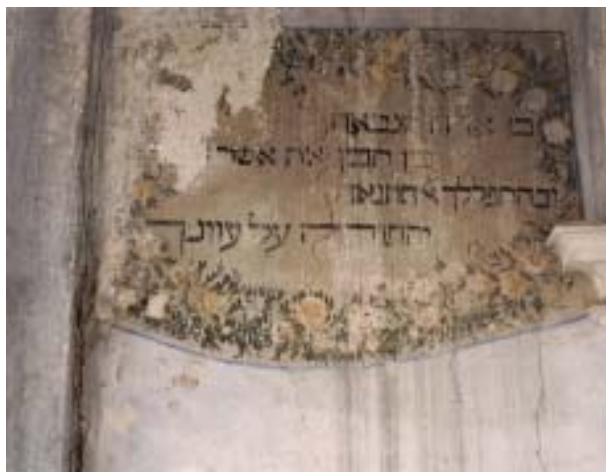
SIGNS OF MOISTURE INFILTRATION
