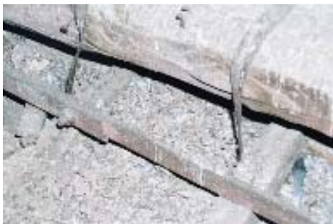
DETAIL OF VAULT REINFORCING
